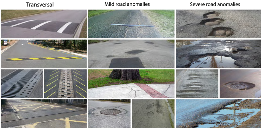
Fig. 3. Types of road anomalies
